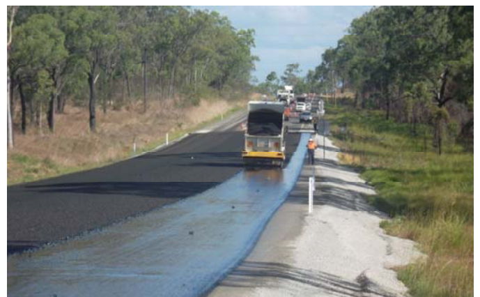
Bruce Highway bitumen works
