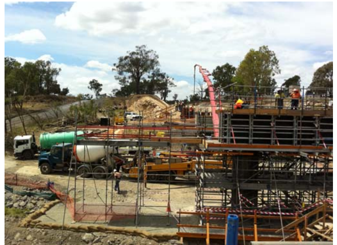
Progress on bridge replacement
